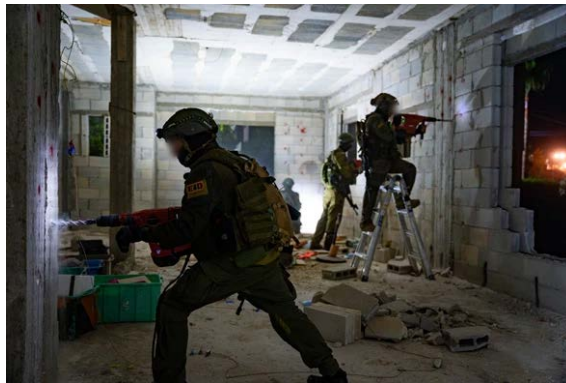
The demolition of the house of Mourad Dahadha (IDF spokesperson, July 31, 2024)
