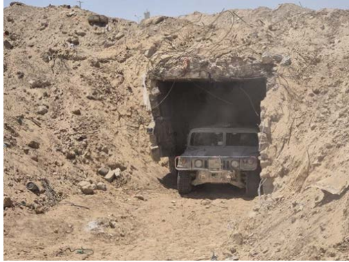
The opening of the tunnel on the Philadelphia Axis (IDF spokesperson, August 4, 2024)
