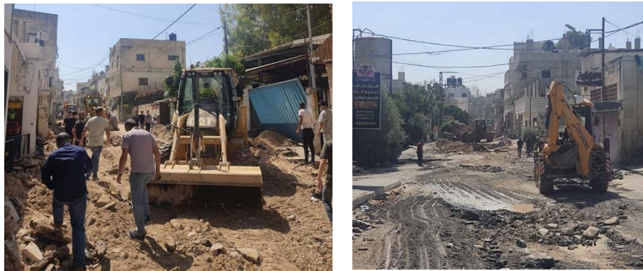
Bulldozers clear the rubble (Wafa, July 5, 2023).
