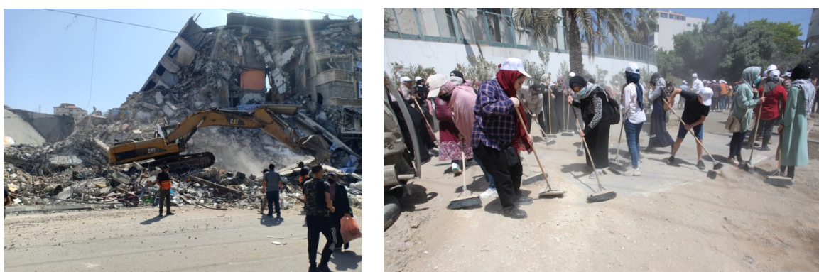
Cleaning the streets and removing rubble (Wafa, May 26 and 29, 2021).
