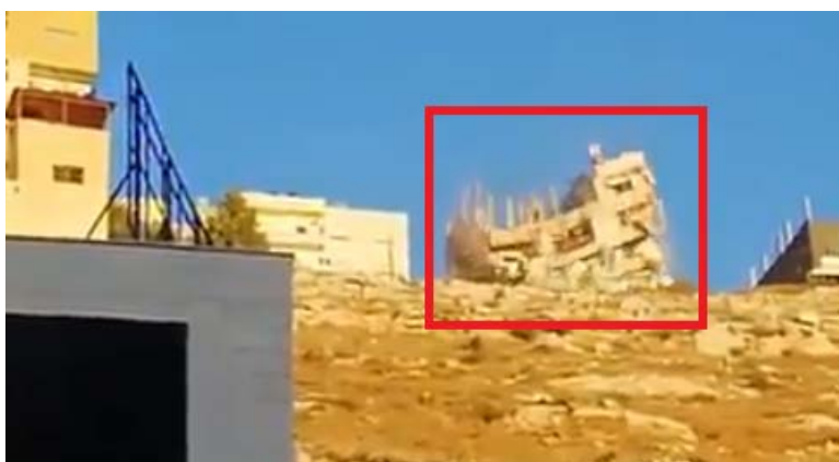
The building after its collapse (aboodrss' Twitter account, August 11, 2018)
