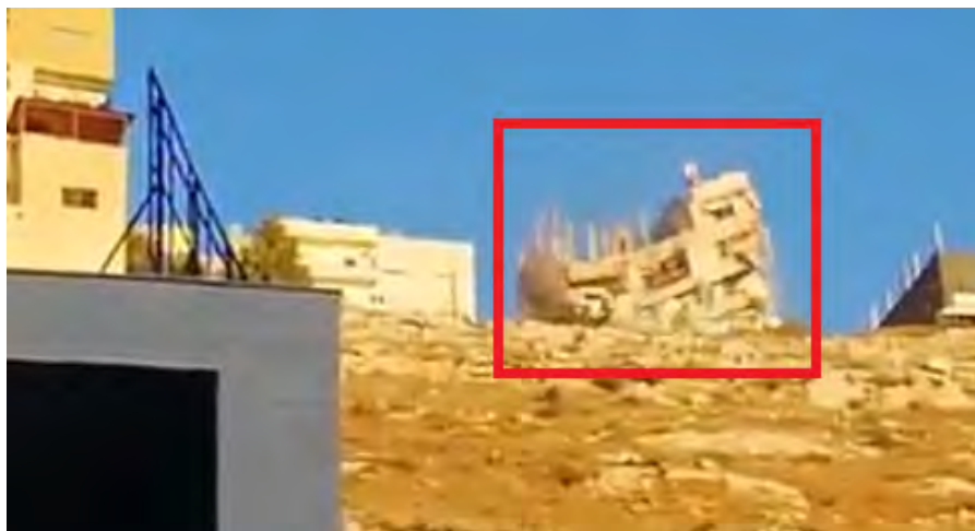
The building after its collapse (Twitter, August 11, 2018)
