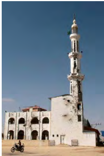
The Ibn Taymiyyah mosque. The damage done during the confrontation, especially to the minaret, is still visible (Reuters, August 16, 2009).
