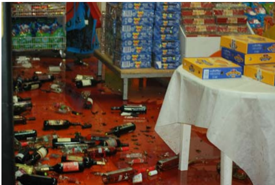
Damage to a store in the commercial center of Sderot caused by rocket fire (Zeev Trachtman, December 17, 2008)
