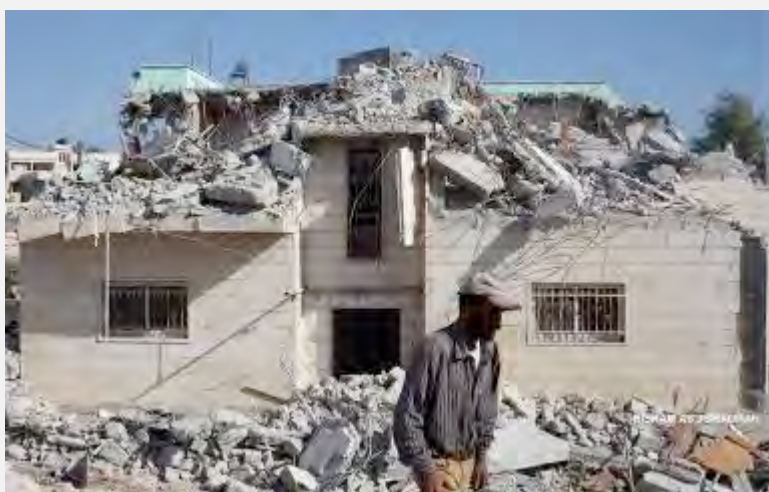
The house of Khaled Makhamra in Yatta after it had been demolished (Facebook page of Shihab, August 4, 2016).
