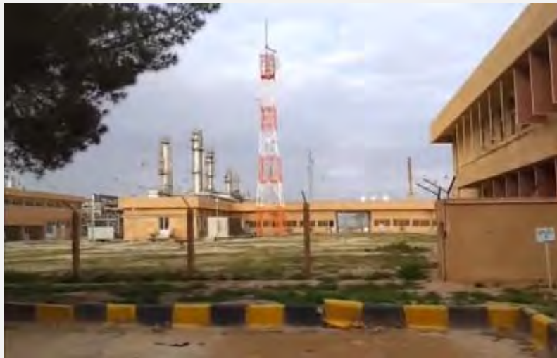
The gas plant in Al-Jabsa (YouTube)
