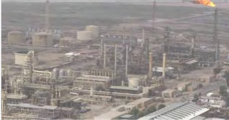
The oil facility in Baiji (Bousla.net)
