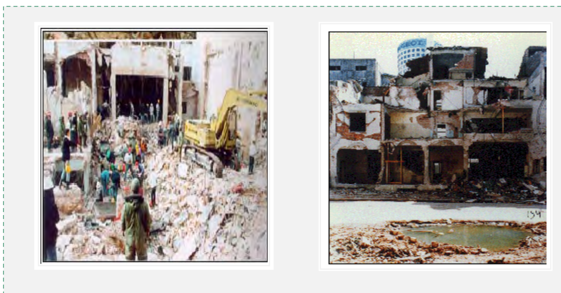
The AMIA building after the explosion. Left: The crater formed by the explosion and the damage done to the building's facade. Right: Evacuating the bodies.
