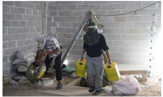
Tunnel opening visible under a tent
